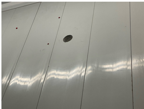
Mini split units were removed
