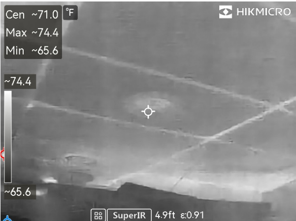
Natural gas system remained cool during heating test
