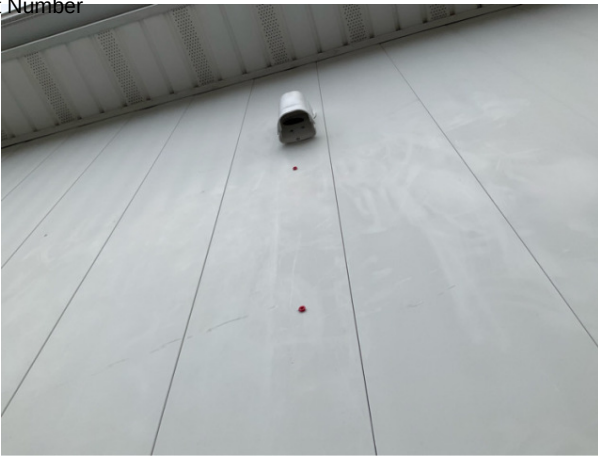
Mini split units were removed and no chases
