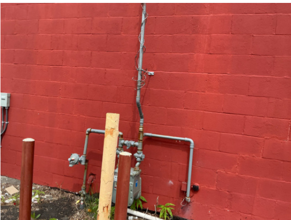
Natural gas line to roof
