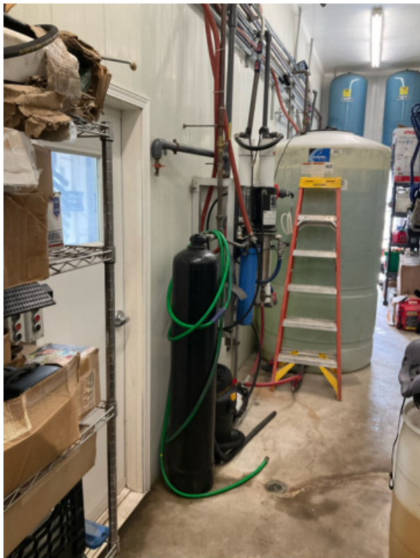
Interior air handler was removed
