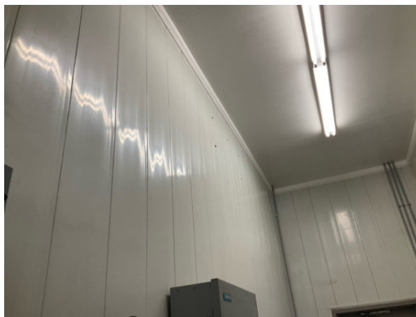
Mini split units were removed
